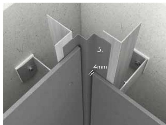
Cembrit Internal Corner is used for 90° internal corners. Secure the profiles with double sided tape. Once fixed, the facade board will secure the profiles in position. There should be a minimum 4mm gap between the board edge and the profile.
