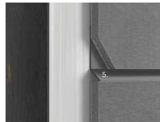
The Horizontal L Profile used for horizontal joints should be cut in the same length as the width of the facade board.
