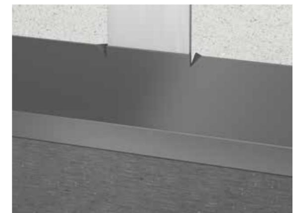
When installing Cembrit vertical profiles, it may be useful to cut and fold out a triangle on each side of the L profile, as shown in the illustration. This will prevent the horizontal profiles (Alu-L profile) from moving.
