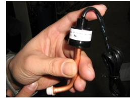
Figure 48: Low pressure sensor.
