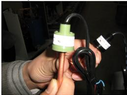
Figure 47: High pressure sensor.
