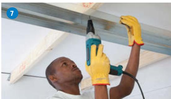
Fasten the top DonnFrame Load Bearing Track at 600mm centres using suitable fixings.
