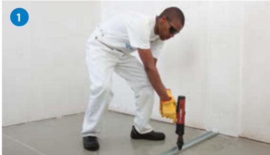
Determine and mark wall position and make allowance for openings. Fix DonnFrame Load Bearing Track at 600mm centres using suitable fixings.
