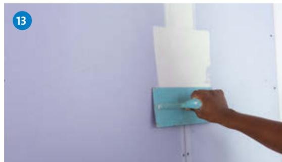
Fill all screw heads and apply a second layer of RhinoGlide using 300mm steel trowel.
