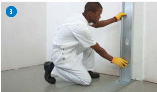
Twist the DonnFrame Load Bearing Stud into place.
