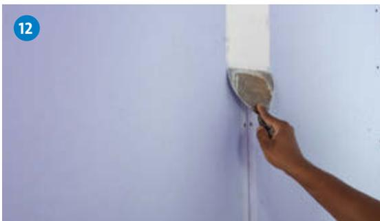
Apply Gyproc RhinoGlide to the joints using a 150mm tapping knife.
