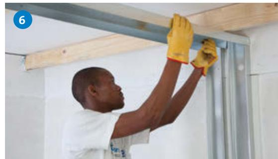
Insert top DonnFrame Load Bearing Stud into position.
