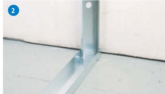
Measure the wall height and cut the DonnFrame Load Bearing Stud to size. Install the stud into the track.
