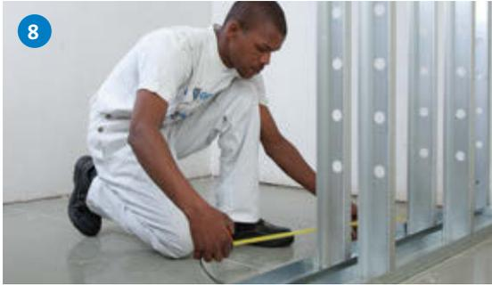
Insert DonnFrame Load Bearing Studs at 600mm centres to a friction fit within the channel sections-this allows for adjustment during boarding. Position the studs so all face the same direction. Apply sealant between the building structure and the framework.
