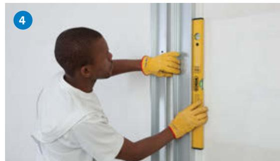
Ensure the stud is plumb and mark stud position.
