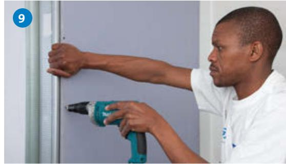
Fix Gyproc SoundBloc to the studs using Gyproc Sharp Point Screws 25mm.
