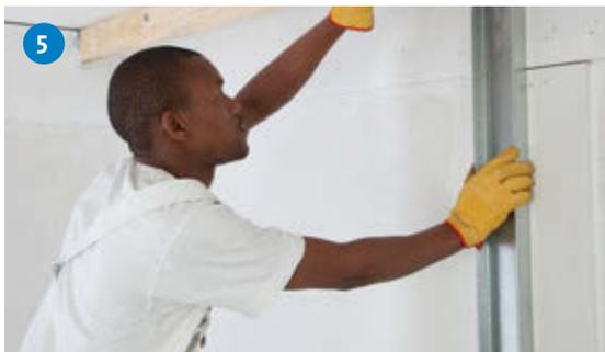
Fix the DonnFrame Load Bearing Stud to the abutting wall at 600mm centres using suitable fixings.
