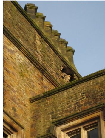
*Dangerous loose masonry to tower*
