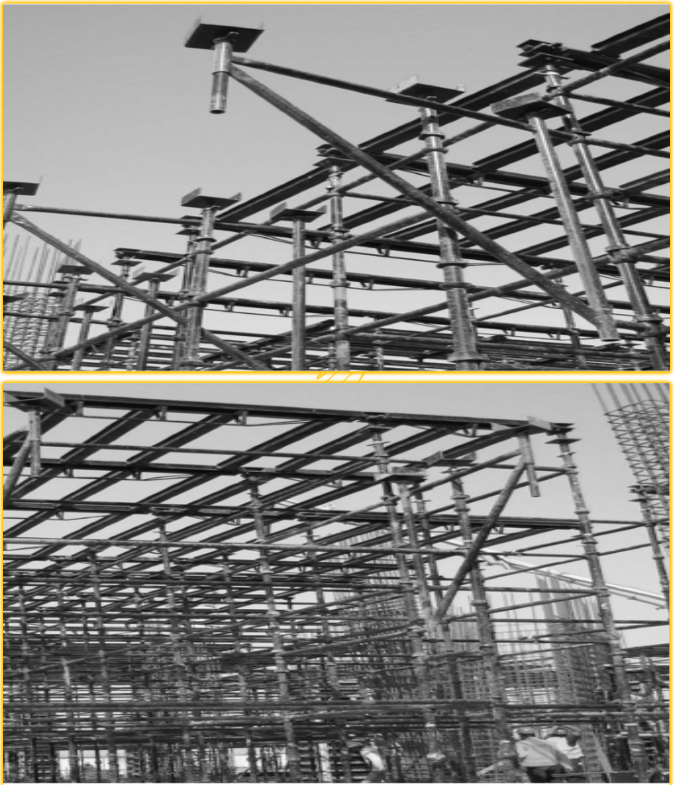
FIGURE 8 DECKING, INFILL BEAMS WITH CANTILEVER &amp; BRACKET BEAMS
