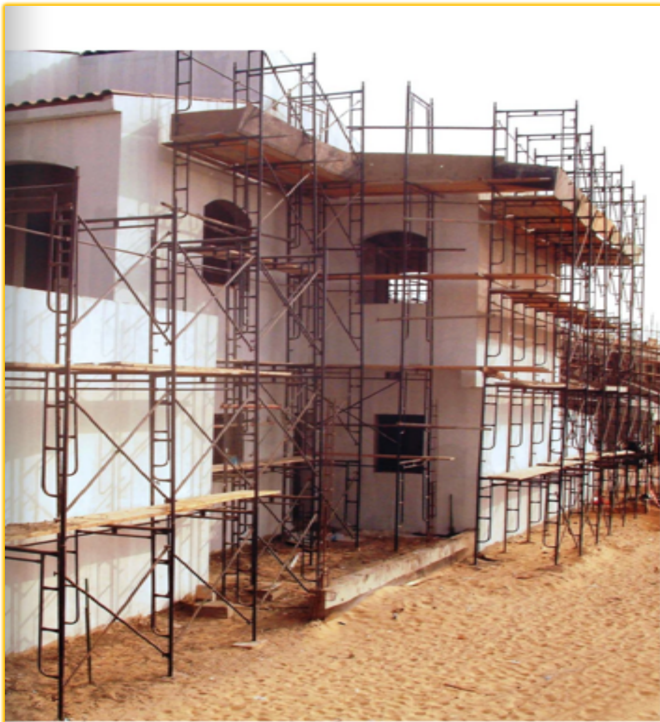
FIGURE 10 HFRAME ON SITE
