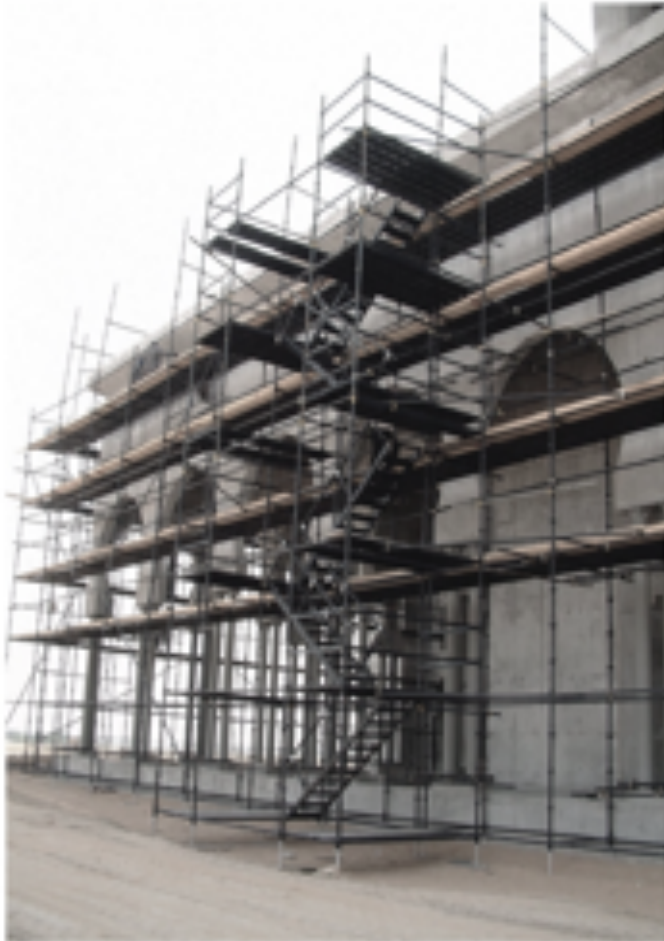
Staircase Tower offers a Full Range of Stairway Solutions for Temporary Access
