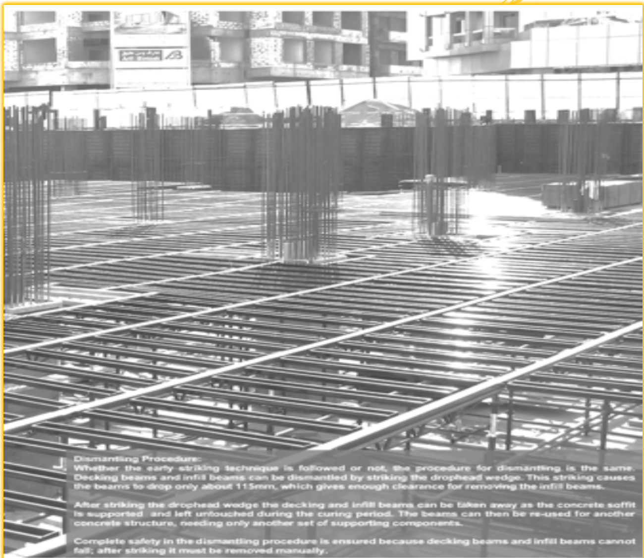
FIGURE 6 CUPLOCK DECKING & INFILL BEAMS OUR PROJECTS
