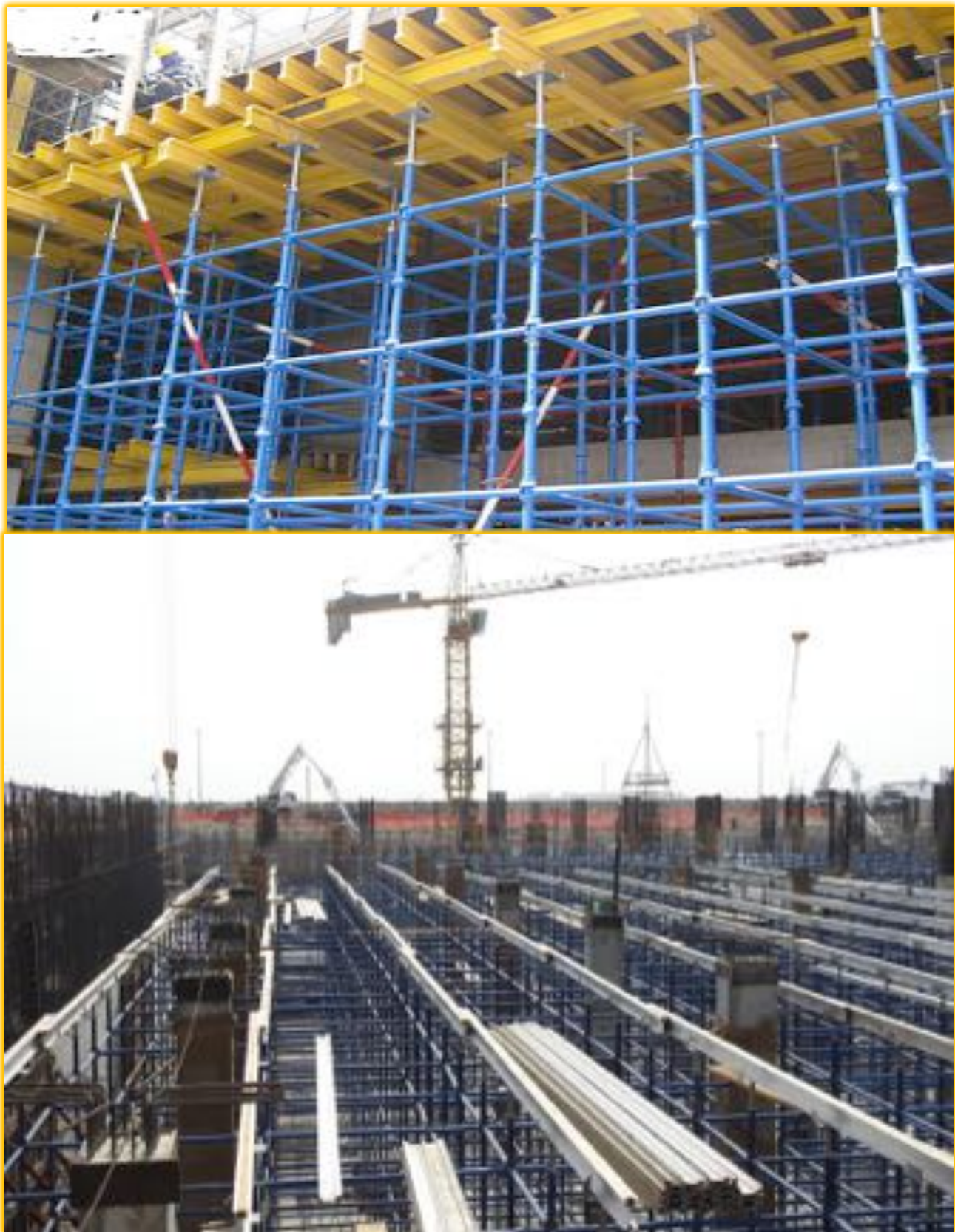
FIGURE 12 CUPLOCK SYSTEM WITH H20 &amp; ALUNINUM BEAMS
